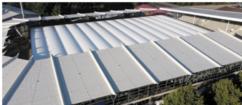
The temporary roof in Stadium 3 at Allianz Park meets the requirements for the vaulting and para-dressage competitions. Photo: ALRV/Saskia Stahl-Farrell
